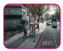
**Floating bus stops** are bus stops that have a road or cycle track going around them, so you need to cross over to get to the bus stop.
